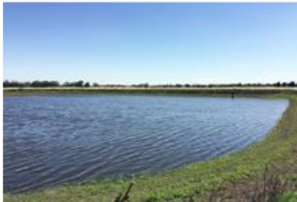
Kagome Australia's reservoir dam
