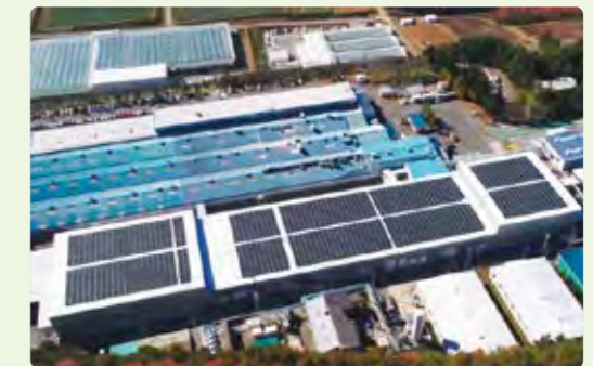
Solar panels installed on the factory roof
